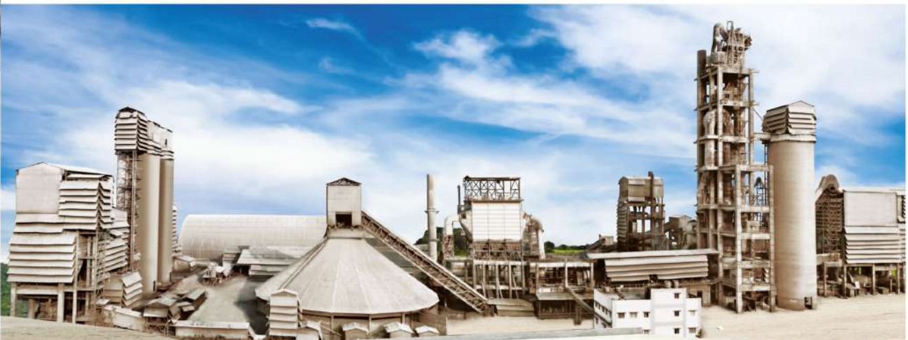
MAX CEMENT INTEGRATED PLANT AT NONGSNING, MEGHALAYA
